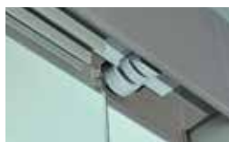
2 Sensors for detector of sash position
