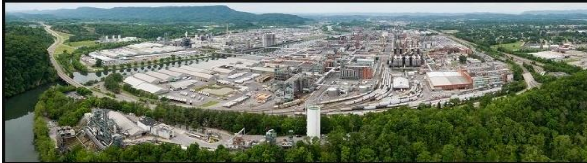
Eastman Chemical Company, Main Site, Kingsport, TN 50 Manufacturing Sites Worldwide, ~14,500 Employees
